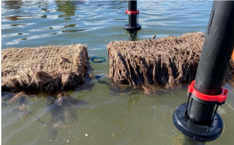
Figure 15 - Jute attenuator with carabiner connections.
