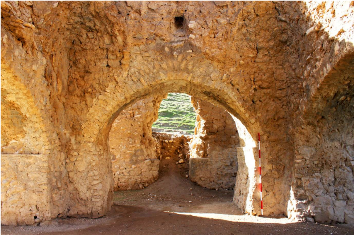
Fig 10. Details of the vaults and the dome
