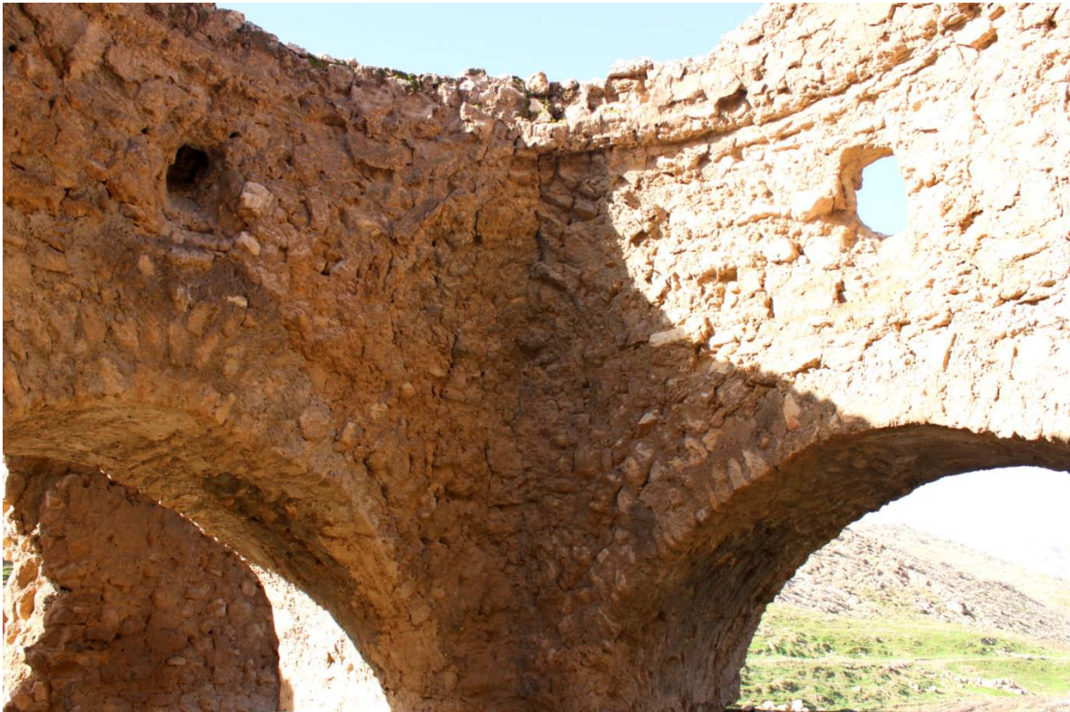
Fig 14. Detail of squinch below the dome
