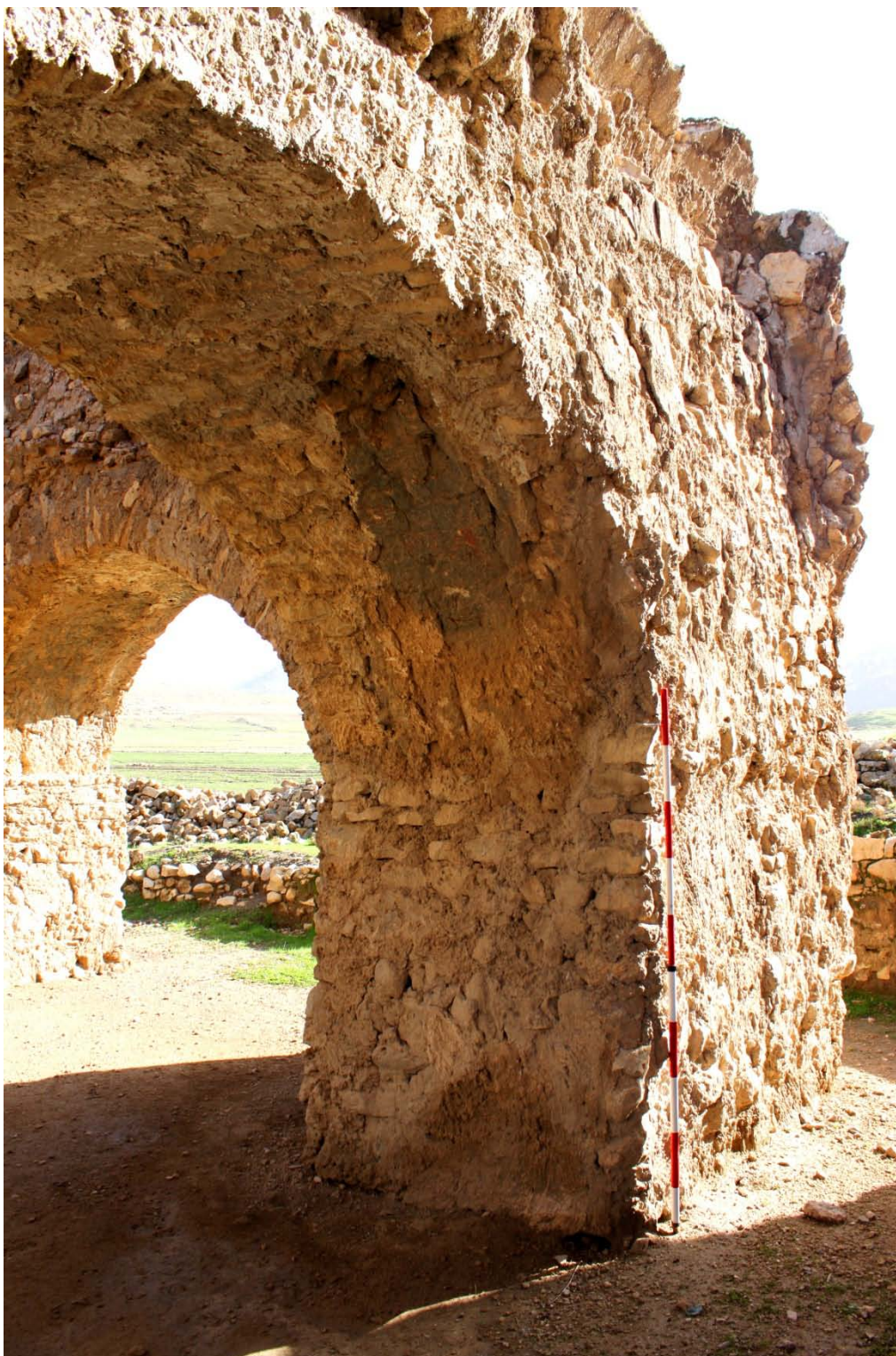
Fig 11. The pillar of the Chahar Taq, southeast.
