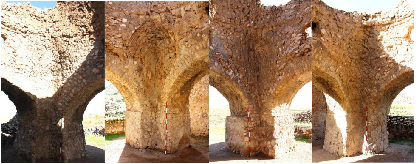
Fig 13. Pillars of the Chahar Taq, view from interior.
