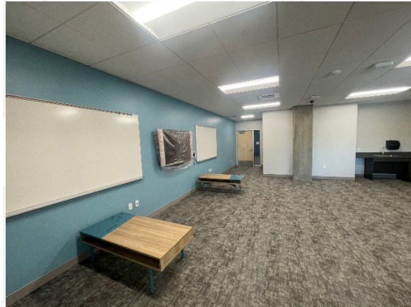
Nursing Simulation Center under construction looking at the Nursing Student Lounge.
