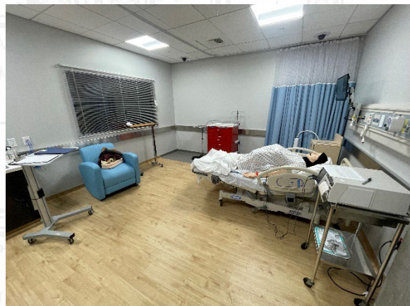
Nursing Simulation Center under construction looking at the OB Simulation Suite at completion.
