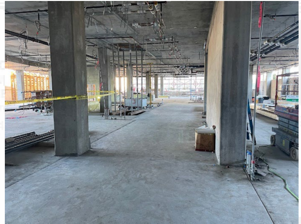
Nursing Simulation Center under construction looking east down the main hallway.
