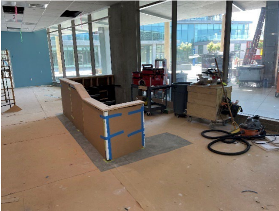
Nursing Simulation Center under construction looking at the Provider Station.
