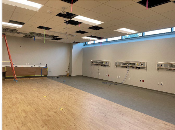
Nursing Simulation Center under construction looking at the Hospital Bed Unit.
