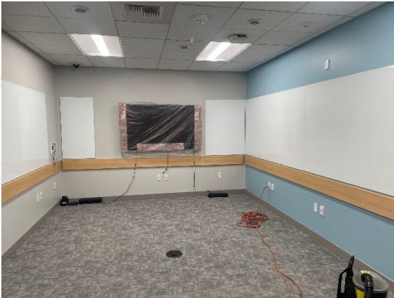
Nursing Simulation Center under construction looking at debriefing room 1.
