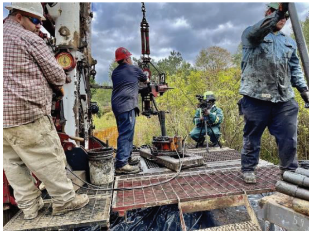
Figure A: WDF plugging an oil well in Bradford Township, PA on Oct. 2, 2021. This well is a legacy well spudded in the late 1800s and was emitting an average of 661 MTCO 2 e/year prior to its plugging.
