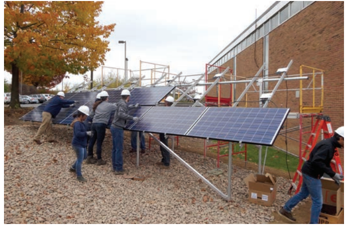
Image 6: Students set 255 W solar panels on array outside of OPP. Credit: Penn State. Creative Commons
