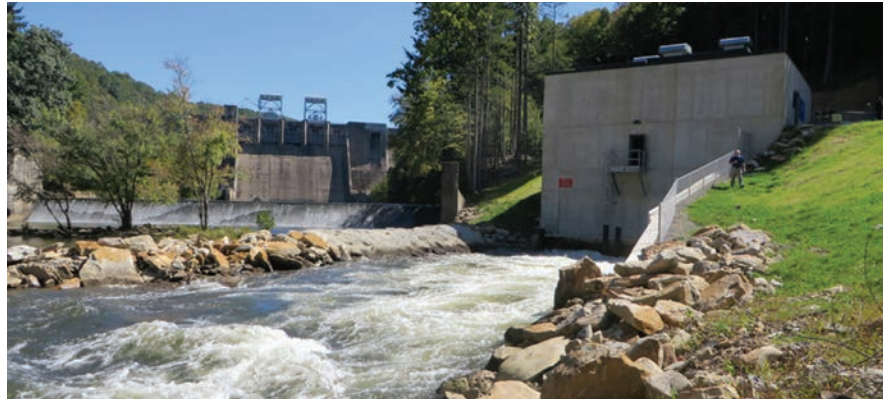
Image 7: Hydro-power dam. Credit: Unknown
