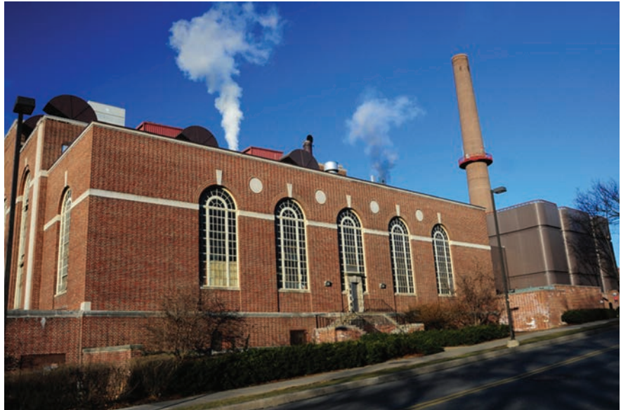
Image 1: West Campus Steam Plant
